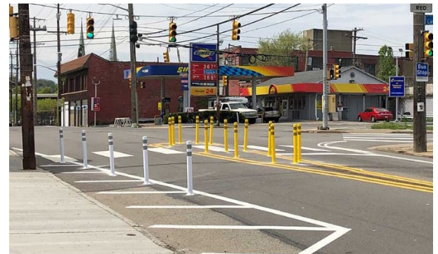
Non-regional (Pittsburgh) example of paint and delineator posts used to provide pedestrian refuge, a shorter pedestrian crossing, and visibility to drivers
