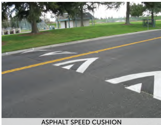
ASPHALT SPEED CUSHION
