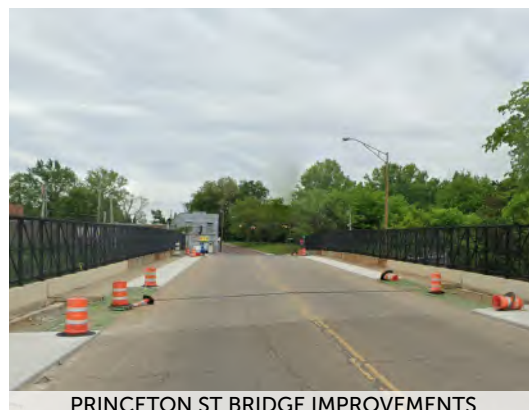
PRINCETON ST BRIDGE IMPROVEMENTS
