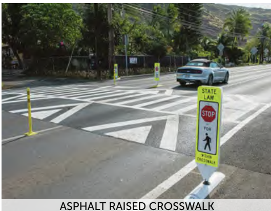
ASPHALT RAISED CROSSWALK
