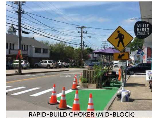
RAPID-BUILD CHOKER (MID-BLOCK)
