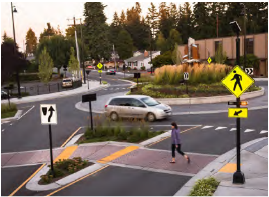
RRFB AT ROUNDABOUT INTERSECTION
