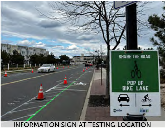
INFORMATION SIGN AT TESTING LOCATION
