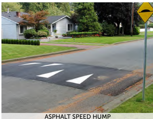
ASPHALT SPEED HUMP
