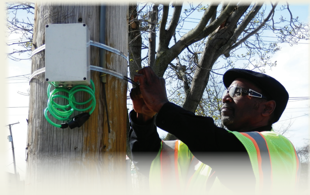
Planning Aide Wali Rahim, setting up one of AMATS' Houston Radar Armadillo Tracker units to collect two-way traffic data.
