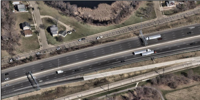
Interstate 76 in Akron, west of SR 59
