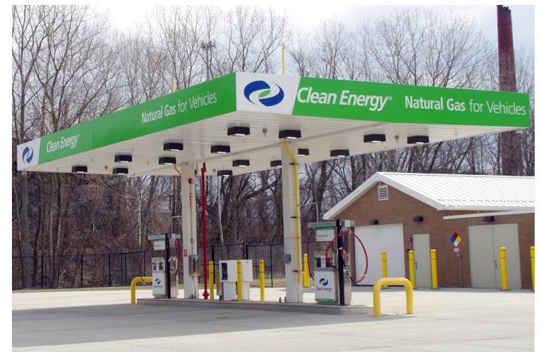
METRO CNG Fueling Station
