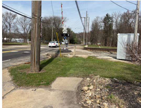
Multiple impediments exist such as the rail crossing along SR-91 which lacks an accessible route
