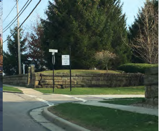
Stone walls in some locations limit sidewalk expansion opportunities.
