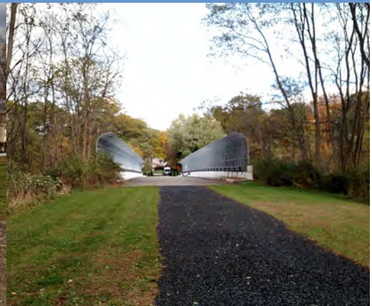
The pedestrian bridge over Interstate 480 connects the west side of the city.
