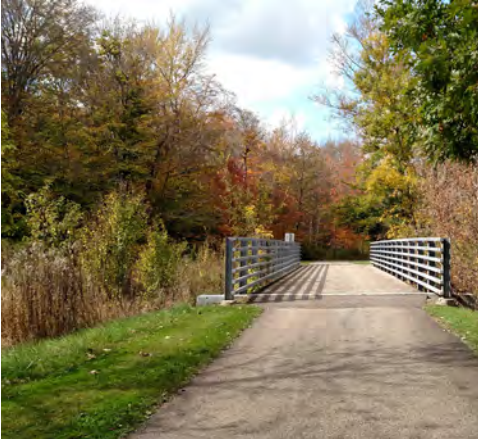
The Center Valley Trail incorporates bridges in a range of locations and styles to provide access across Tinker's Creek.
