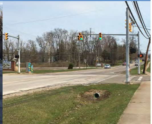
Intersection at school entry drives - safer crossing details are needed.
