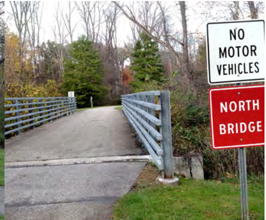
Bridges throughout the system traverse scenic Tinker’s Creek.
