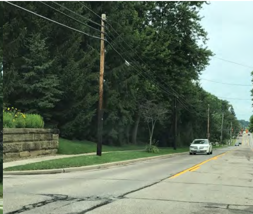
Wide lanes promote higher speeds along corridor.
