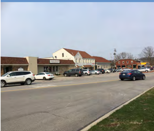
A parking zone in front of commercial uses creates unusual patterns of vehicular movement.
