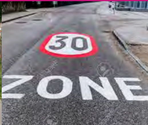
Pavement markings for speed reduction
